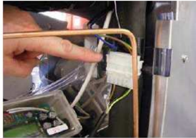
3. Disconnect the cable to the agitator motor
